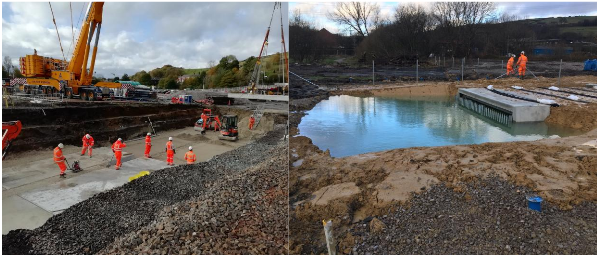
Figure 10: Photos of the box culvert during construction (left), and after construction when the dewatering system was turned off and the groundwater level had rebounded (right).
