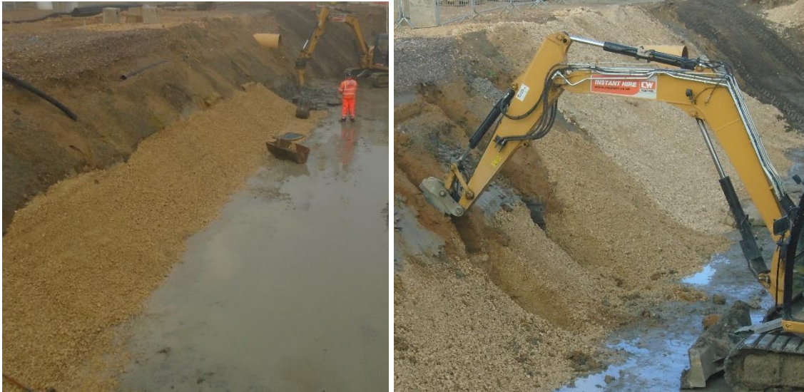
Figure 9. Construction of angular stone key. Figure. 10. Construction of aggregate wedge
