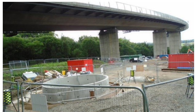
Figure 5. Photo of micro-tunnel reception shaft located close to the bridge piers.
