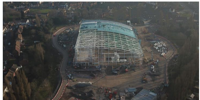
Figure 11. The Birmingham Commonwealth Games Aquatic Centre during construction.
