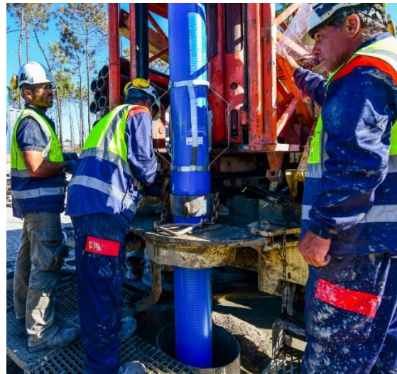
Figure 9. Drilling of deep dewatering borehole.
