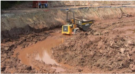
Figure 1. A site without any groundwater control.
