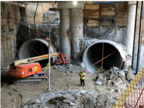
Figure 15. Drawdown achieved beneath the metro station.
