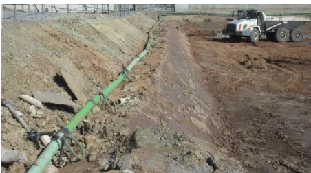
Figure 2. A site with appropriate groundwater control.
