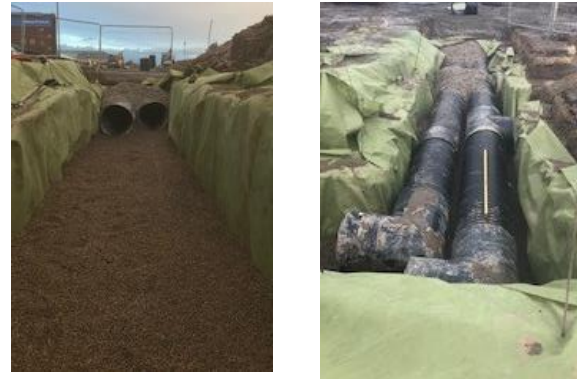
Figure 5. Perforated pipes within attenuation trenches.
