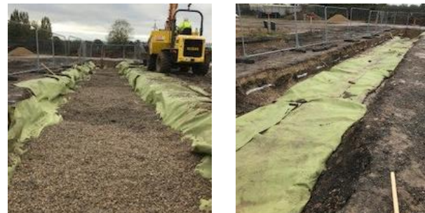
Figure 6. Final backfilling of attenuation trench and wrapping with green nonwoven geotextile.
