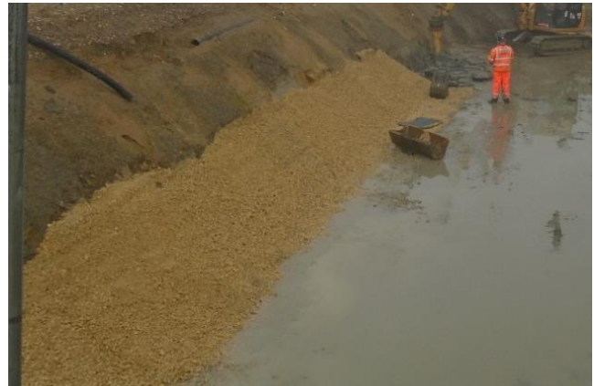
Figure 9. Construction of angular stone key.
