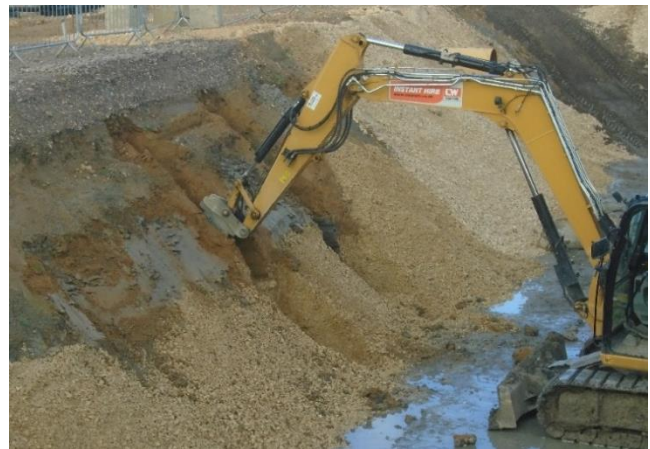
Figure 10. Construction of aggregate wedge.
